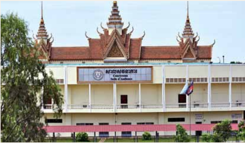
The courthouse of the ECCC
