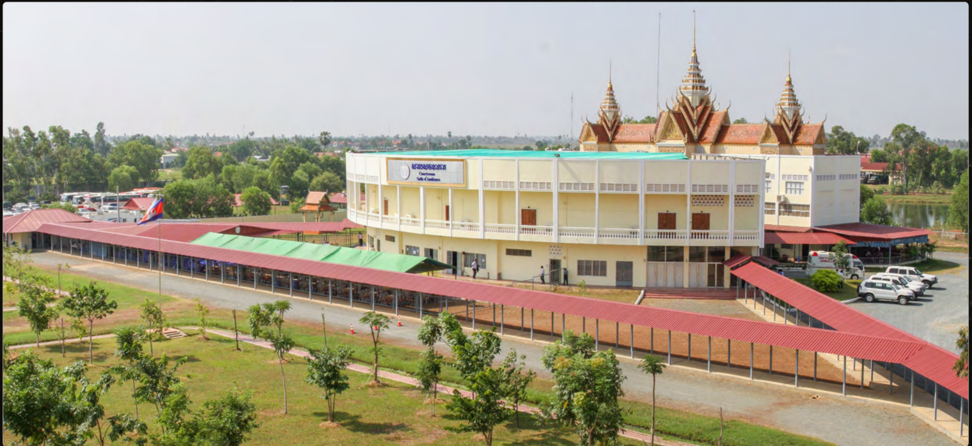
The ECCC Courtroom building, located in Choam Chao on the outskirts of Phnom Penh.
